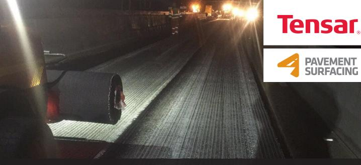
Tensar's Glasstex P100 increased pavement strength and mitigated reflective cracking.
