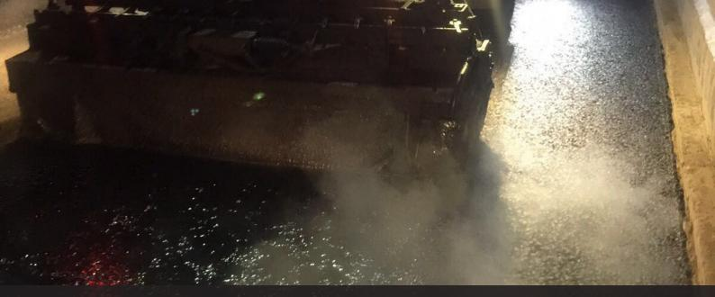
Glasstex adhered to the underlying pavement structure using a bitumen bond coat.
