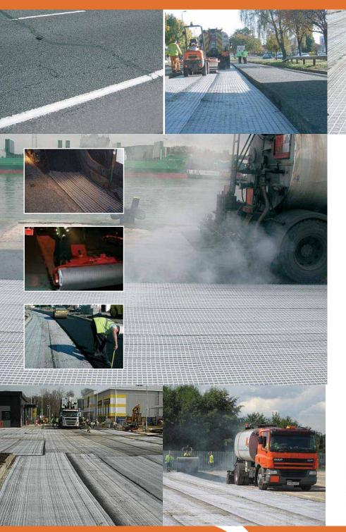
FCL are suppliers and installers of geosynthetics and composites for asphalt overlay. We use our own calibrated binder distributors to spray a bond coat of 160/220PEN (straight run) bitumen. The hot applied binder is compatible with all asphalts and requires NO BREAK TIME.
