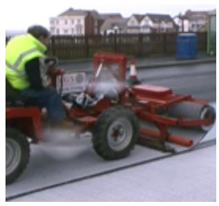
The existing asphalt was milled off to a depth of 50mm and a pre-regulated asphalt surface 25mm thick was placed. 200 pen bitumen spray was then applied and 11,000 m2 of Glasstex® P100 was installed using a purpose built lay-down machine for speed and accuracy by specialist installer AGS Ltd, now operating as Foster Contracting Ltd. A 14mm stone mastic asphalt (SMA), 40mm thick surfacing course was then placed directly on to the Glasstex®.
