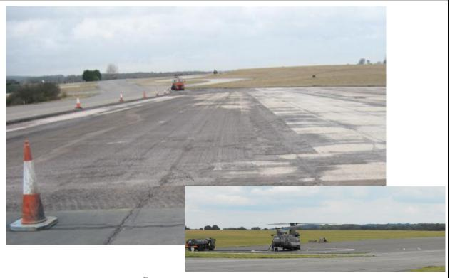
Centre: Overlay milled-off ready for Glasstex® installation. Right: Repaired airfield for Chinook helicopters
