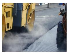
Surfacing is placed directly on Glasstex<sup>®</sup>
