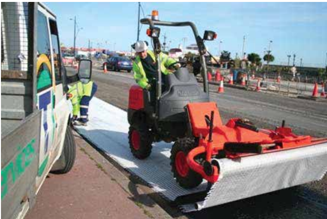
Installation of the geosynthetic
