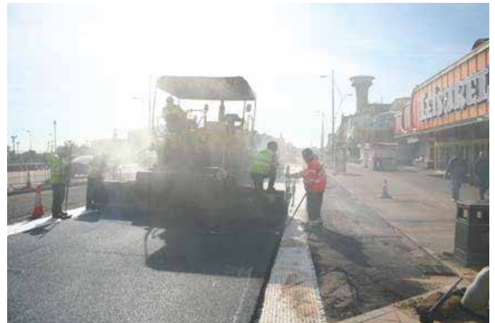
Installation of the Polymer modified surface course
