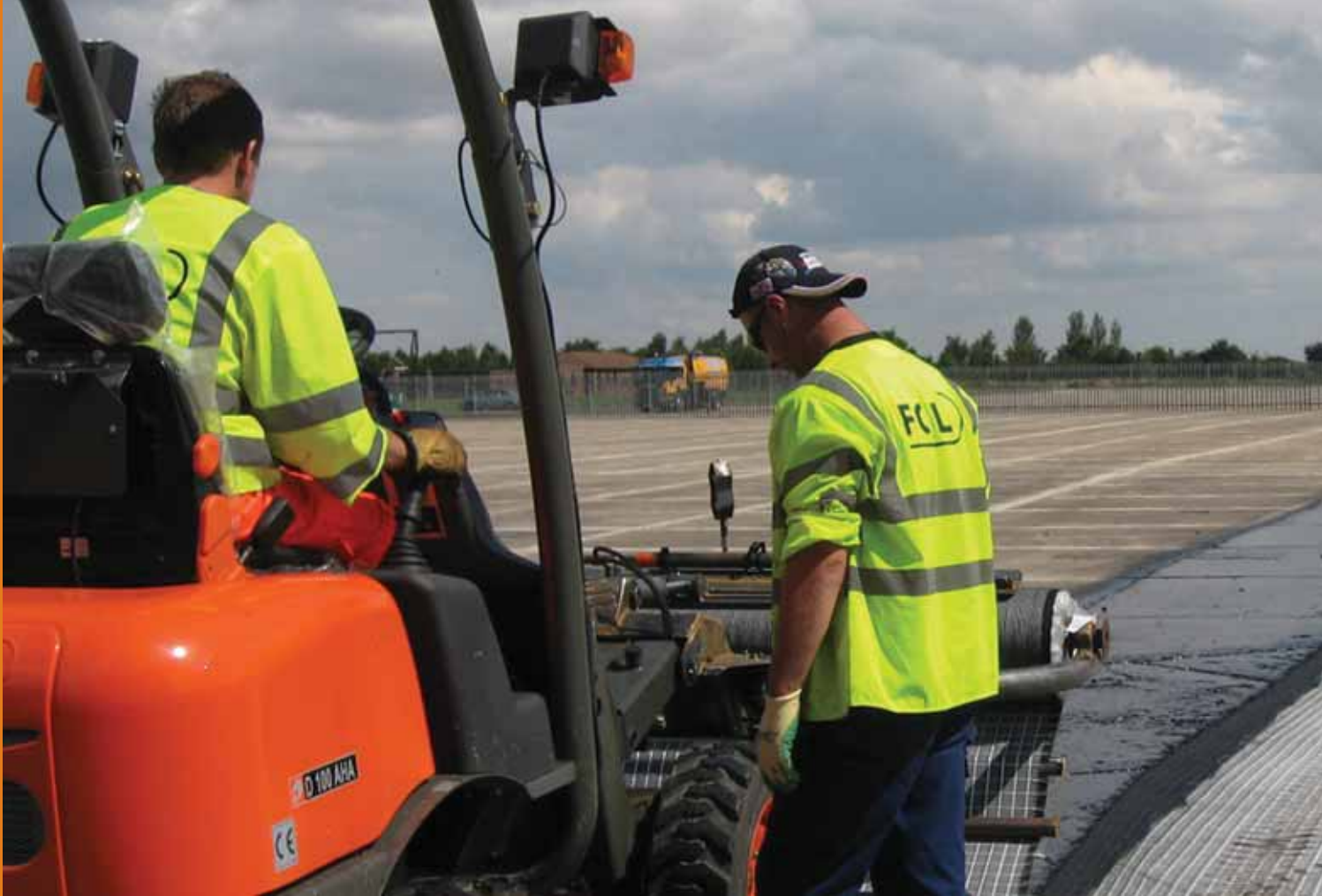
Tensor asphalt reinforcement systems can be used over concrete to mitigate reflective cracking problems
