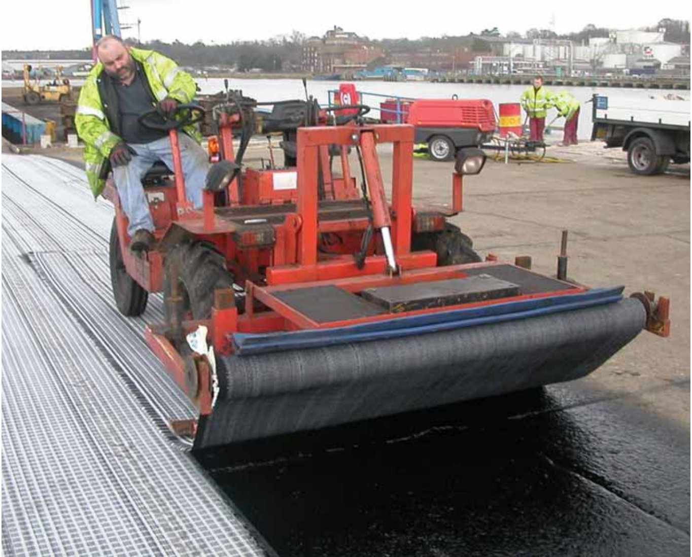
Glasstex® and Glasstex® Grid can be used to control reflective cracking in thinner surfacing layers
