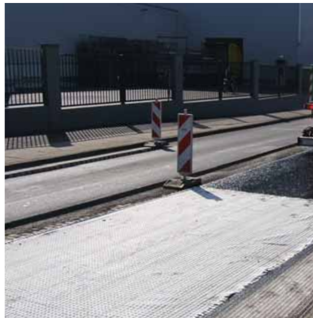
A simple overlap joint for Glasstex®
