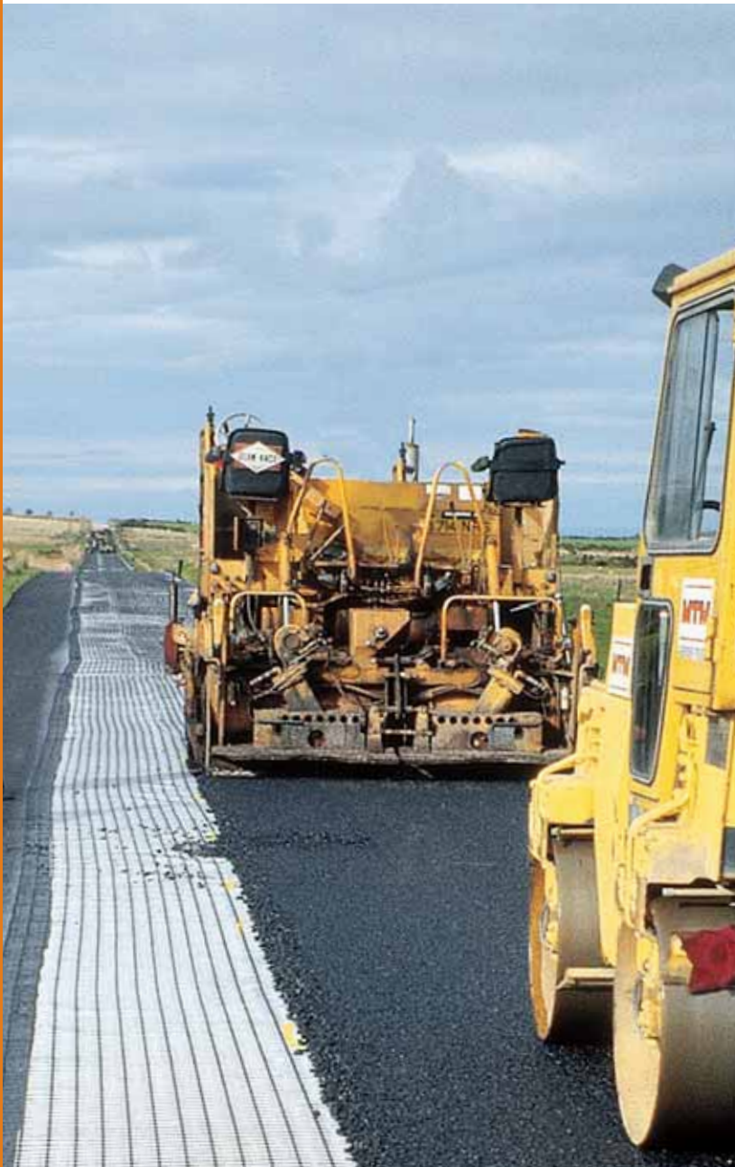
Tensor AR-G bonds well into the underlying surface to allow paving directly over the grid
