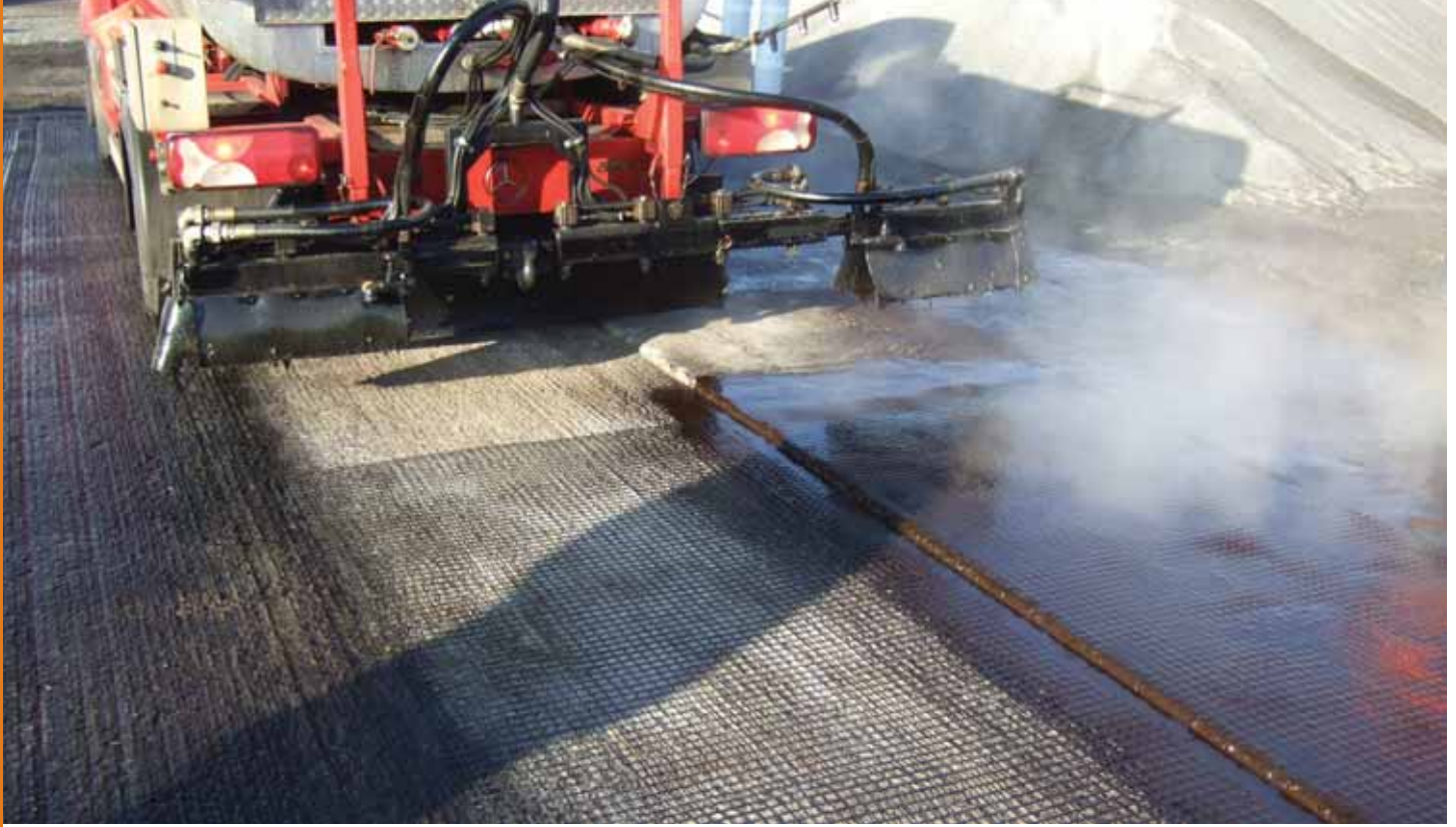
Glasstex® Grid has a self-adhesive coating on the underside to secure the grid before paving
