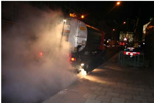
Spraying of the bond coat
