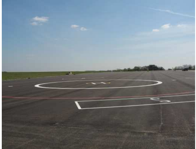
The completed helicopter airfield
