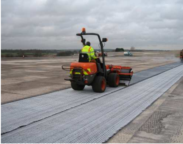
Rapid mechanical installation of Glasstex
