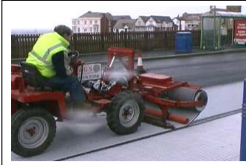
Glasstex is rapidly machine installed
