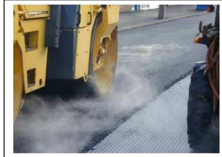
Surfacing is placed directly on Glasstex
