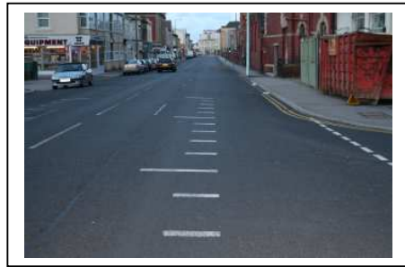
No sign of cracking after 8 years in service
