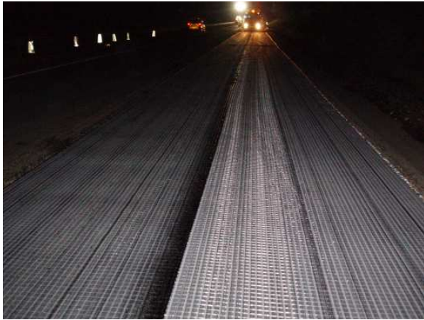
Glasstex is bonded onto the planed surface
