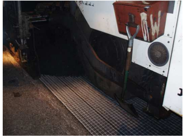
Binder course placed directly onto Glasstex
