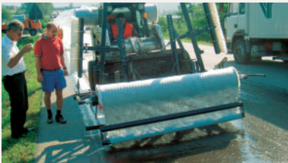
Geosynthetic installation with TenCate laying equipment.
