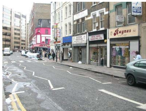
View of the road surface : 2007
