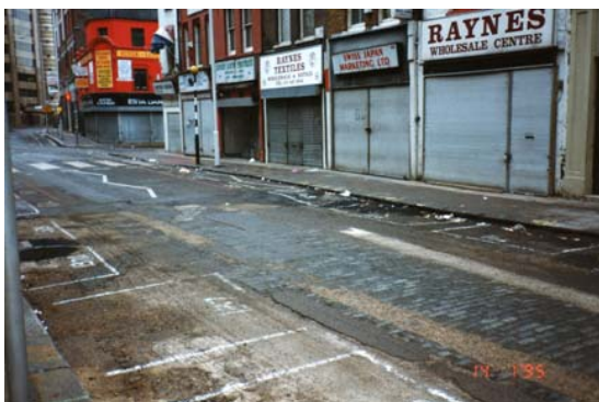
View of the existing road surface : 1995
