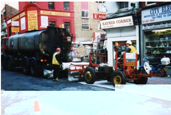
Installation of the PGM-G 100/100
