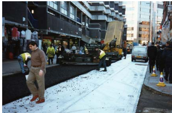
Installation of the PGM-G 100/100
