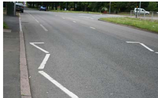
No sign of cracking after 8 years in service
