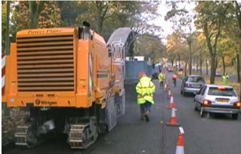
Old asphalt is planed off
