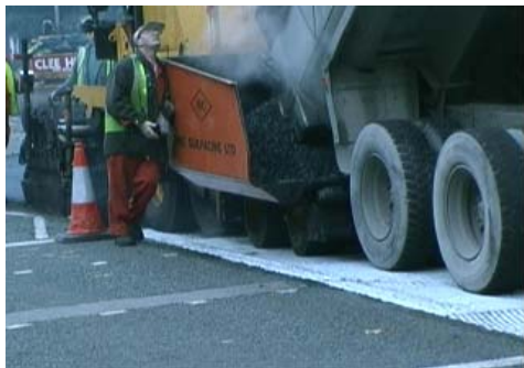
Paving directly on to the Glasstex
