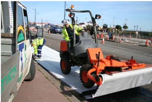
Installation of the PGM-G 100/100
