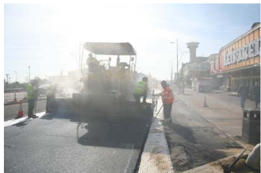
Installation of the Polymer modified surface course
