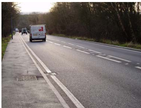
The refurbished carriageway
